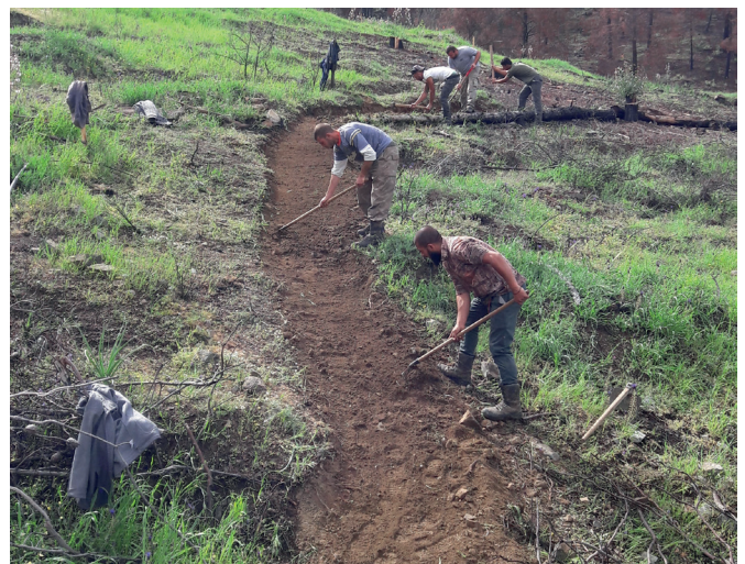
Constructing the path at Karterouni (Erin Gibson)
