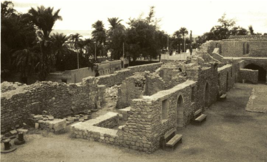
Aqaba Castle: The west range, as rebuilt following destruction by naval bombardment in 1912 and 1916–1917
