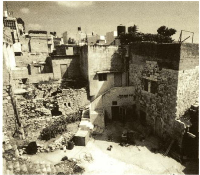
Courtyard of Bayt Hawain looking north-east
