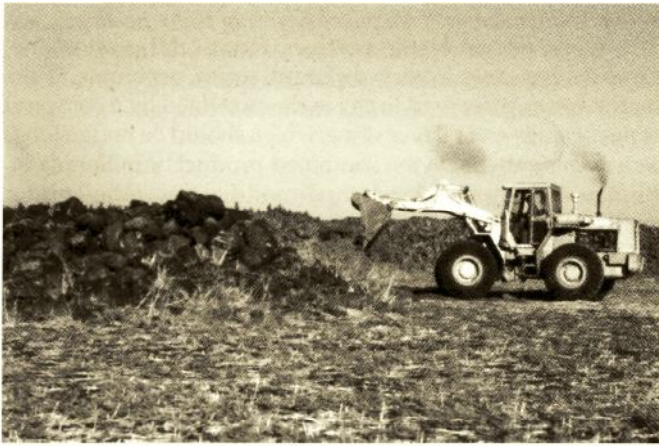
Bulldozer destroying ancient cairns and field systems adjacent to one of the project's test areas
