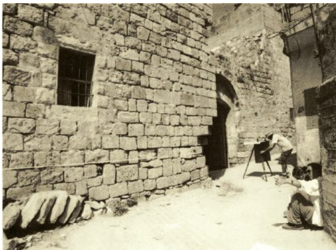
Main (east) facade of Bayt Hawain showing crown of vault projecting above ground at the foot of the wall on the left, and main entrance on right. Note the adjustment in the lower courses of masonry to accommodate the earlier vault
