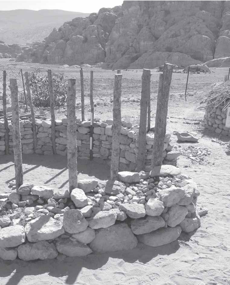
Experimental Building 48 under construction
